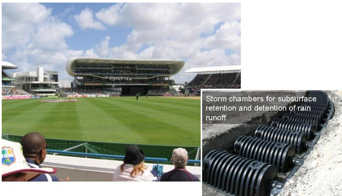
Figure 7: Storm water retention and infiltration at the cricket stadium in Barbados.
