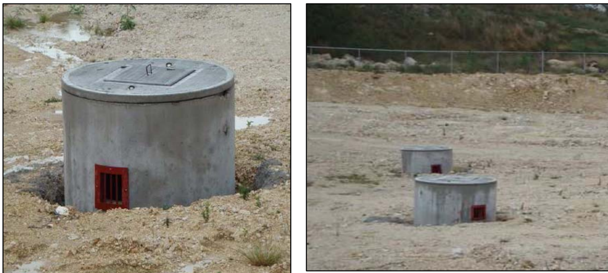
Figure 8: Suckwells located in an infiltration basin for storm runoff, Barbados. Source, Smikle and Yokon, 2008.
