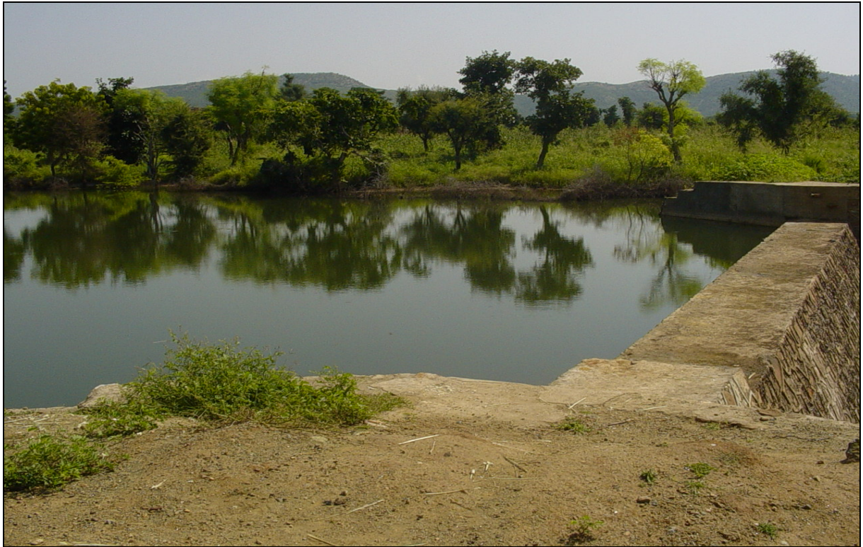
Figure 10: Masonry check dam in Rhajasthan, spillway elevation 2m.
